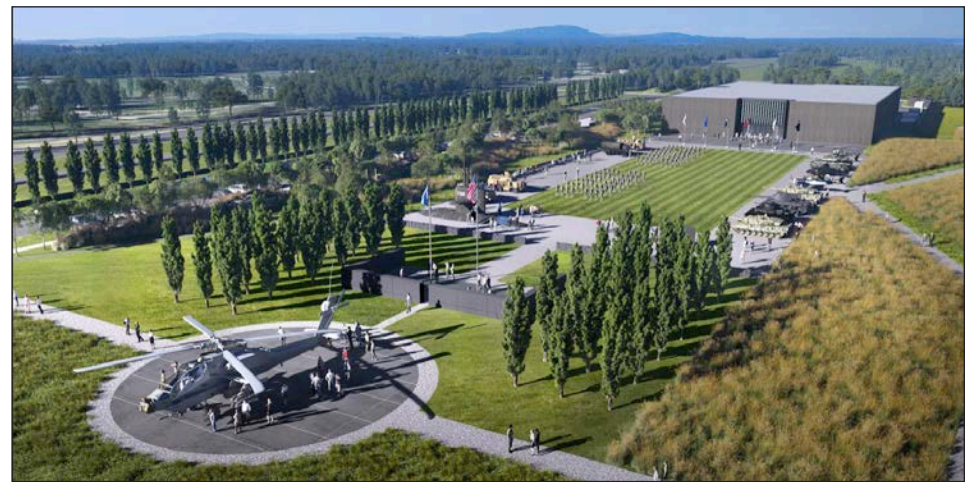
Here is an aerial view rendering of the future Minnesota Military & Veterans Museum. The $33 million project is expected to break ground this spring, with a tentative grand opening in 2025.
