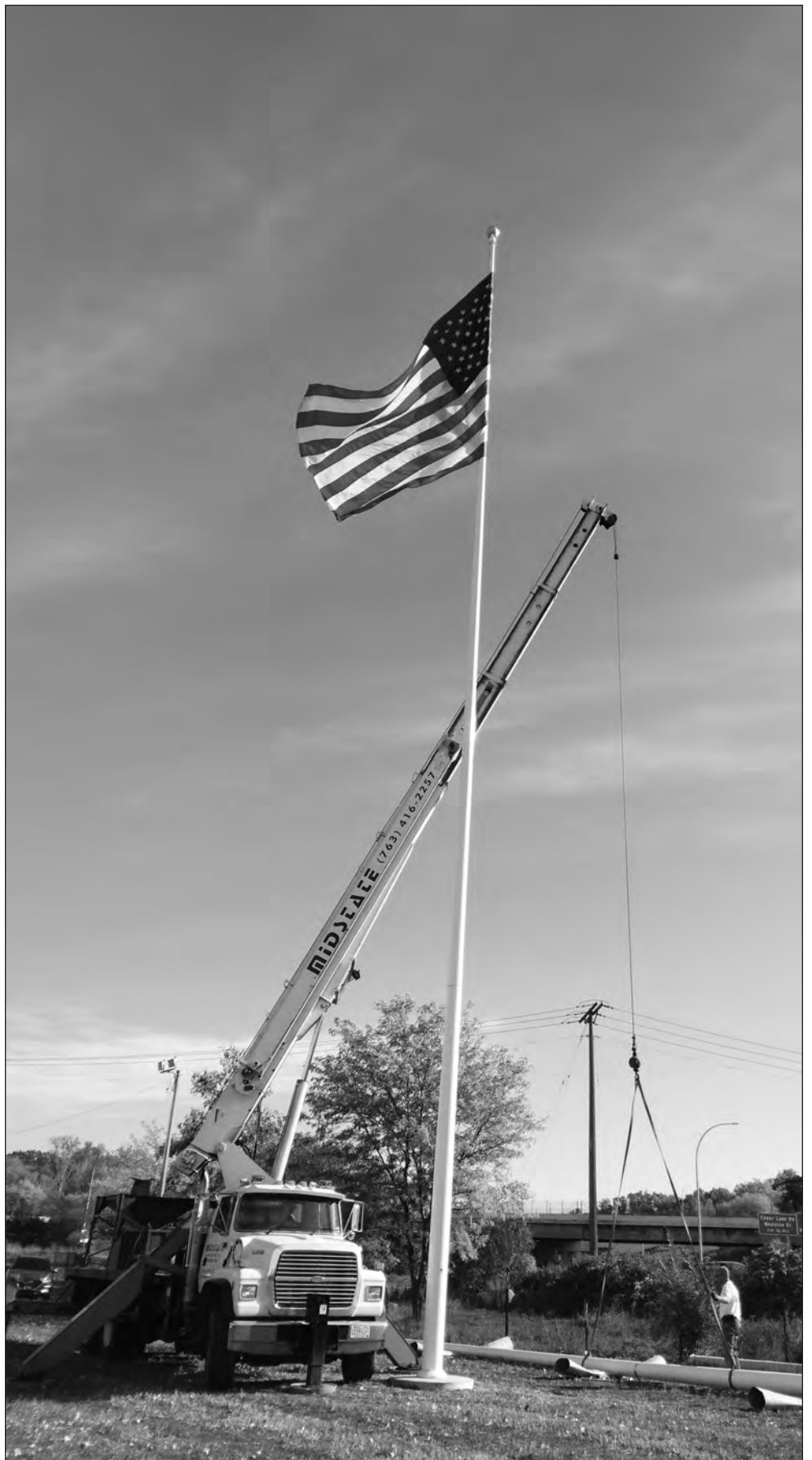
Golden Valley Post 523, better known by its tribute name of "Chester Bird," erected a new flagpole near the end of September. It was totally funded by member donations. The pole is 80 feet tall. The concrete footing weighs 14,500 pounds. The flag is sited prominently on Minnesota Highway 100 at the edge of our parking lot. "We wanted to let everyone driving by to know who we are, where we are and what we stand for," said Commaner Craig Hartman.
